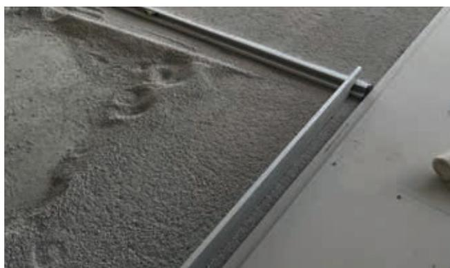
2. Pose des plaques types fermacell 25 mm.
